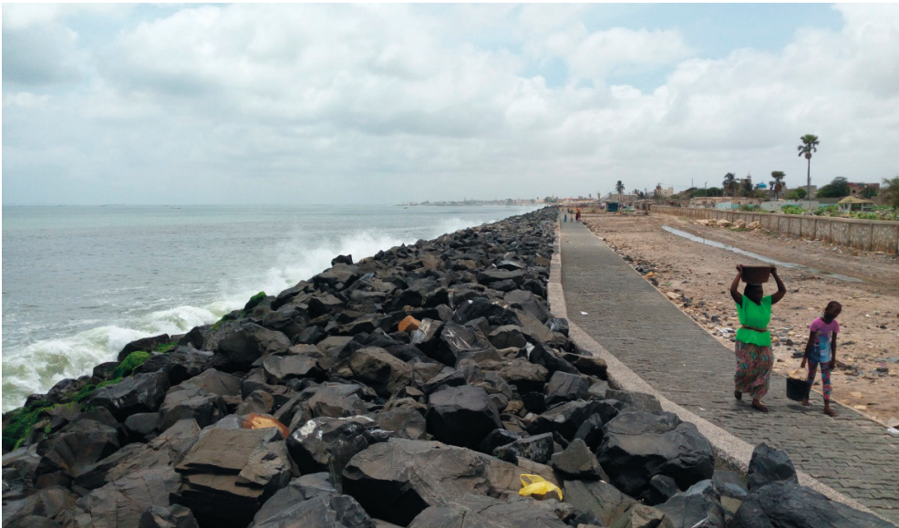
Fig. 16. The Frontal Dyke of Thiawlene (Rufisque) (author's field visit – August 2020)
