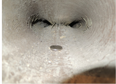
Fig. 7. Inner profile of crushed string after spherical cap - spherical cap rams have been used
