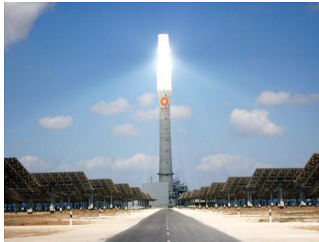
Figure 11. Example of solar tower with receiver.
