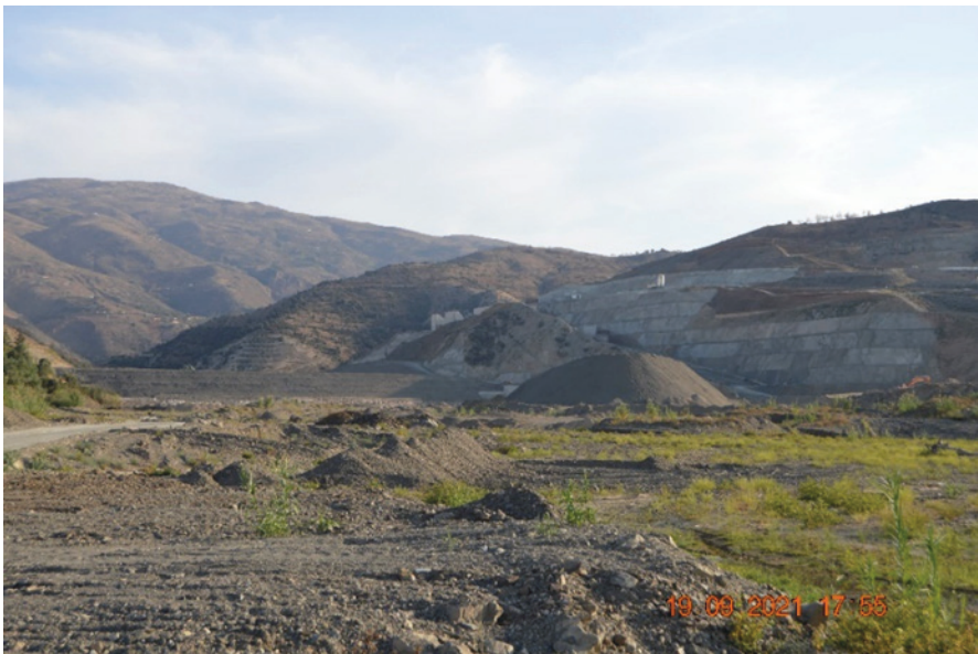
Fig. 2. Dam under construction in the Ghiss basin
