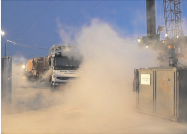
Fig. 3. Preparation of foam cement with N_2
