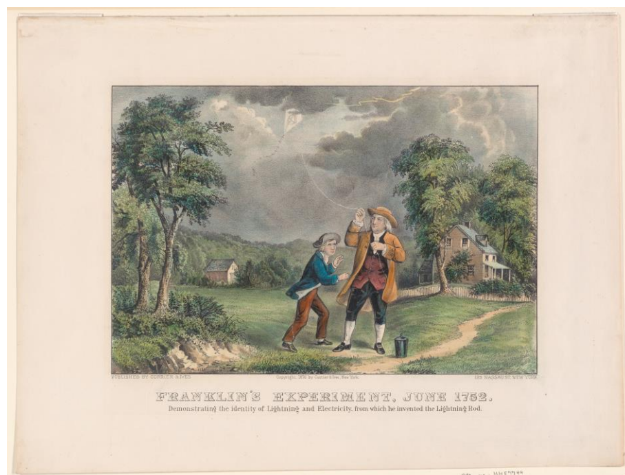
Fig. 2-3. Franklin’s kite experiment, identifying the lightning and electricity [37].
